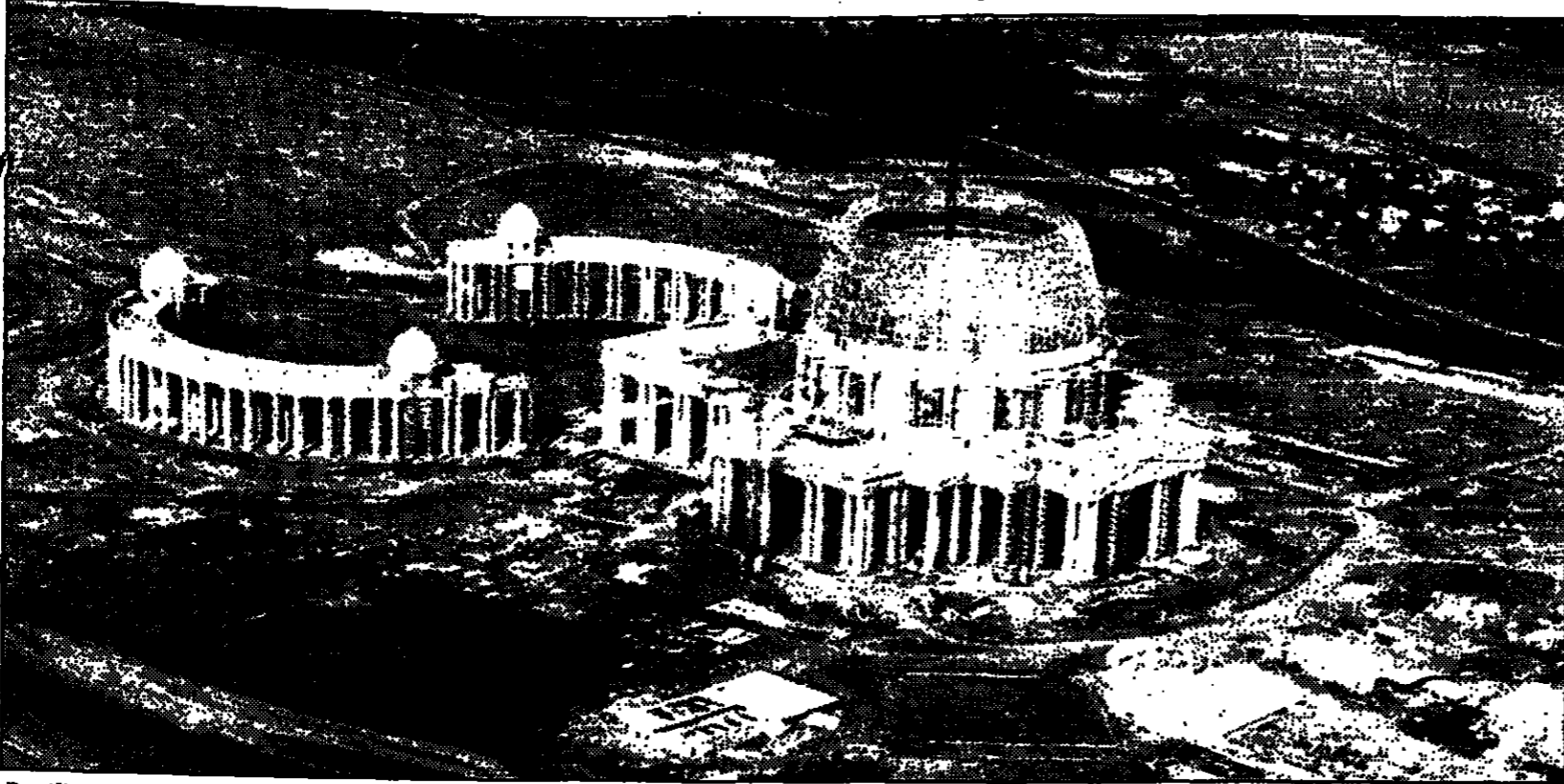
Basilica, planned to be world's largest, under construction in Yamoussoukro.
